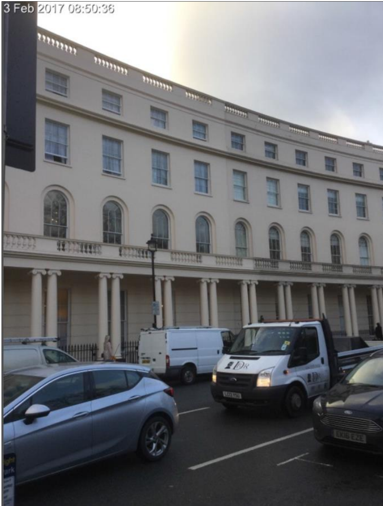
Site 2 7-8 Park Crescent W1
